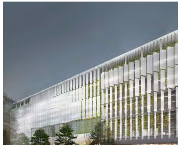
Bagley Parking Hub, Detroit
